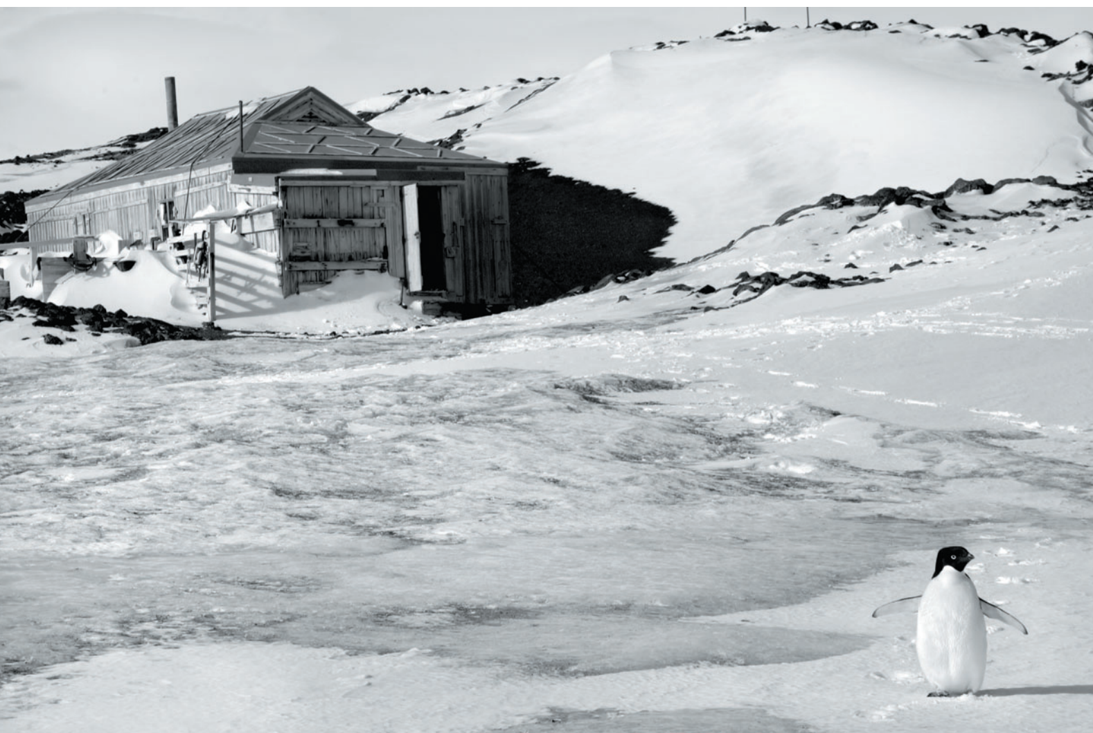
BELOW Cape Royd's hut built by Shackleton and his crew in 1909
